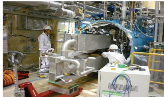
图3 日本J-PARC低温系统因油污染进行检修照片 Fig. 3 Overhaul of J-PARC cryogenic system due to oil pollution in Japan
